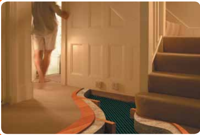
Insulation installed between wooden floor joists
