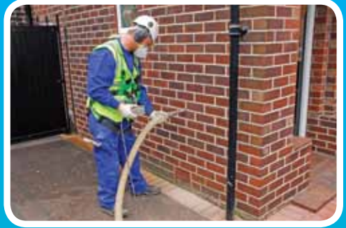
Cavity wall insulation being installed by a qualified professional
