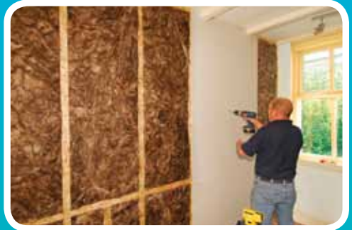
Internal wall insulation being installed in a terraced home
